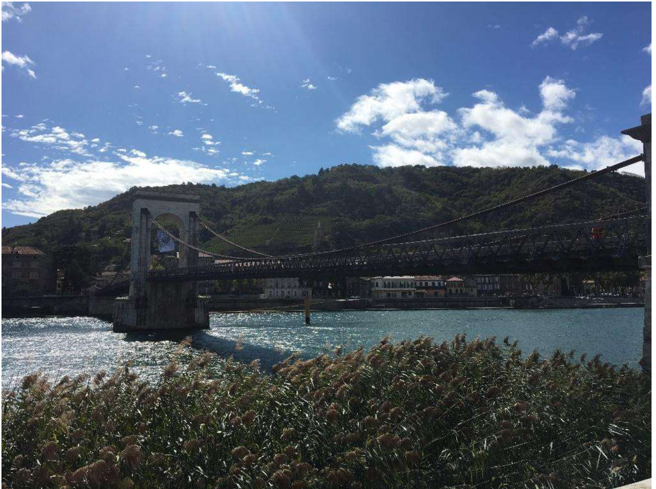
The bridge across the Rhône at Tain
